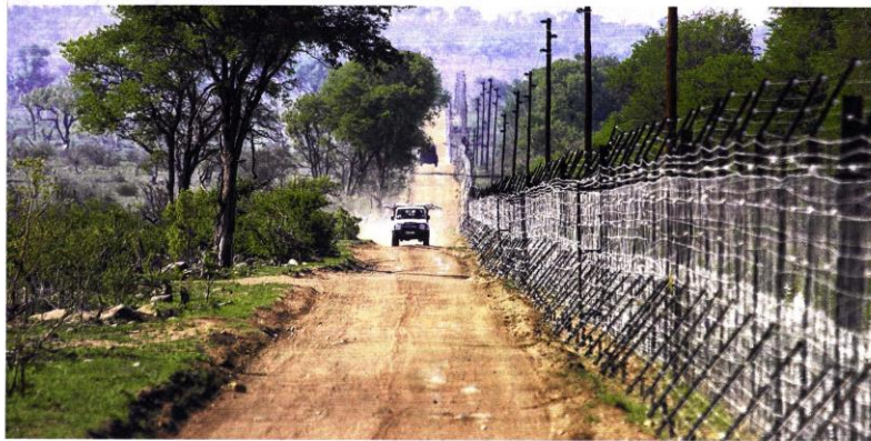
A patrol car driving by a fence which separates a private game reserve in South Africa from neighbouring farmlands and homes. The fence has sensors which alert rangers to any breaches. It is part of a pilot programme using technology to ward off poachers. ST PHOTOS LIM YONG
